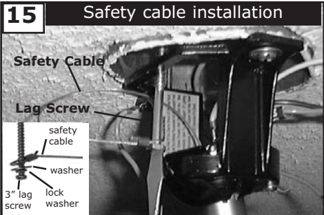
15 Safety cable installation Fan and light kit combinations over 35 lbs, in both flush and downrod mode the safety cable must be installed into the house structure beams using the 3" lag screws, washers, and lock washers, provided. Make sure that when the safety cable is fully extended the lead wires are longer than the cable and no stress is placed on the lead wires.
